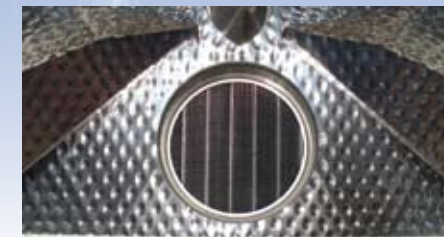
Water-cooled heat exchanger installed
